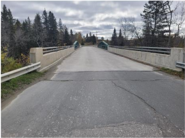
1. North Approach (looking south)
