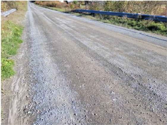
3. Wearing Surface (looking east)
