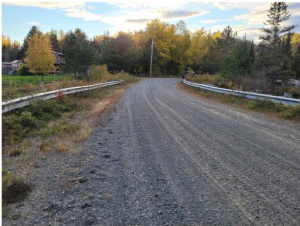
1. East Approach (looking west)
