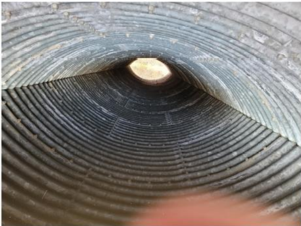
6. Inside Barrel (looking north)
