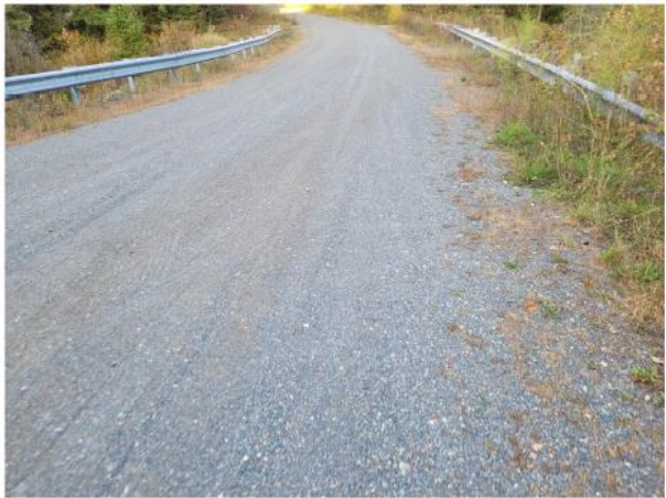
3. Wearing Surface (looking east)
