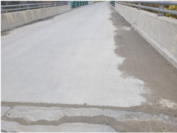
3. Wearing Surface (looking north)
