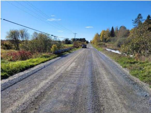
1. East Approach (looking west)
