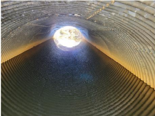
5. Inside Barrel (looking south)
