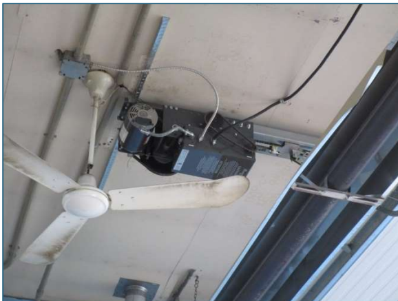
Picture 15 - Tight ceiling clearance between fan, door opener and heater at Markstay Hall
