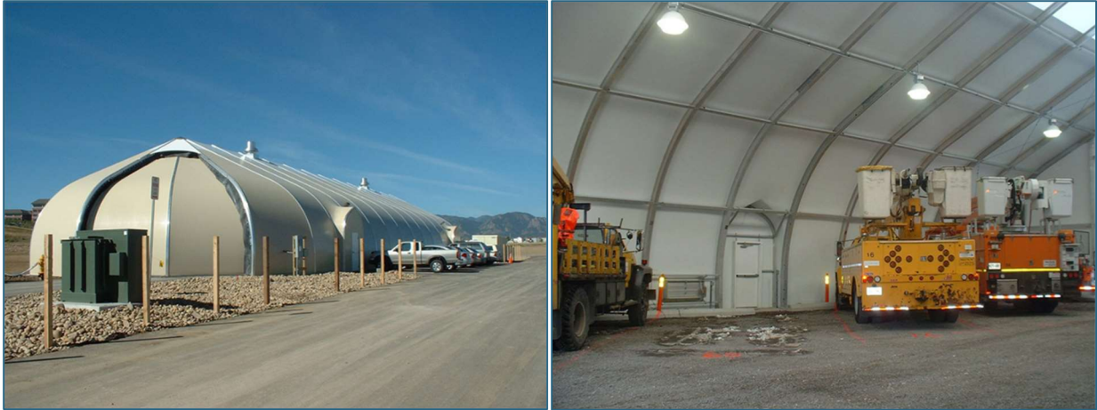
Picture 19 - Example of a Public Works Yard with Membrane Construction
